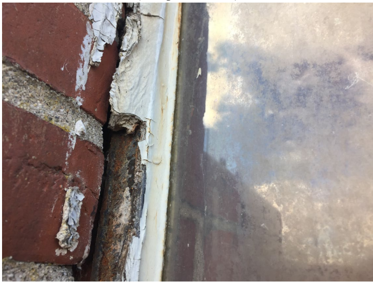
Closer view of ACM caulk on Units 3&4 windows, east side
