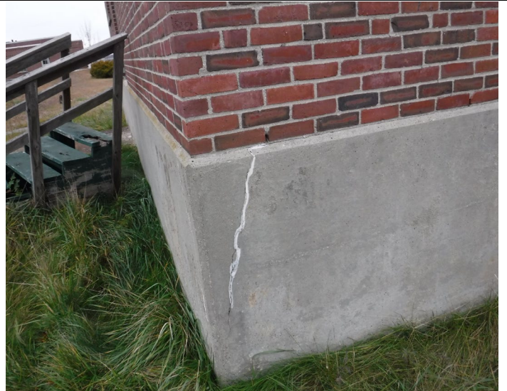
Closer view of ACM caulk on Screen House 3 exterior foundation
