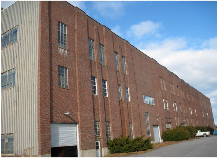
View of the front (east) elevation of the Powerhouse Building. View is to the northwest.
