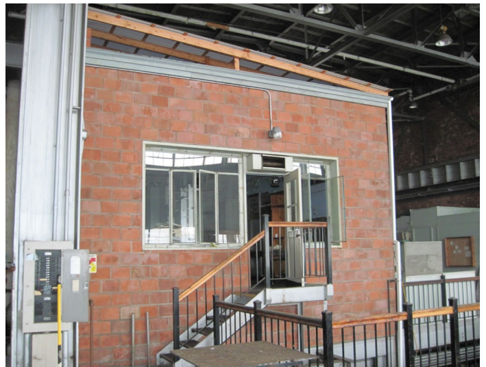
View of former CMP Control Room, located on the third floor
