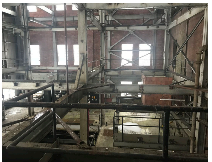
Unit #5 Area of Powerhouse building, previously cleared of large-unit equipment, piping, and most ACM.
