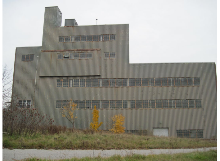
View of the south elevation of the Powerhouse Building. View is to the north.
