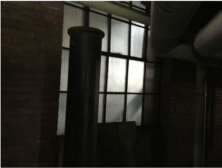
All steel-sash windows have ACM glazing, building wide, including interior windows “trapped” by subsequent additions.
