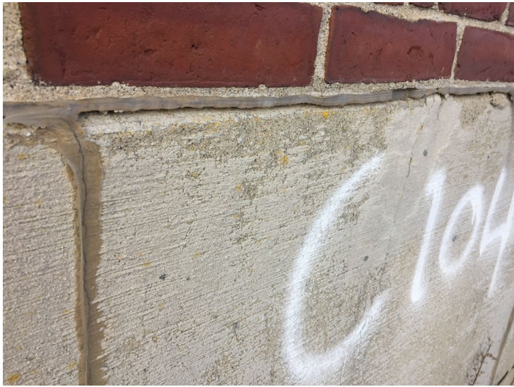
ACM caulk on Units 3&4 concrete foundation (Sample set C-04)
