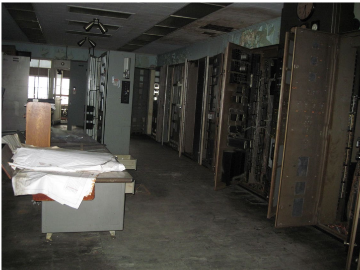
Interior view of former CMP Control Room
