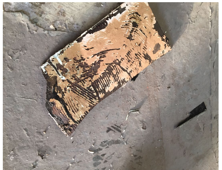
ACM mastic on vinyl covebase, CMP Control Room interior (Sample set 06)
