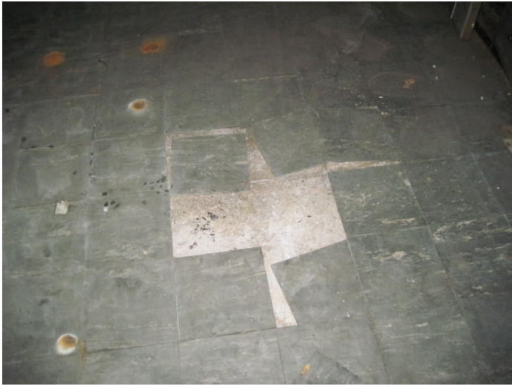
Floor tile with ACM mastic, CMP control room interior (Sample set 07)
