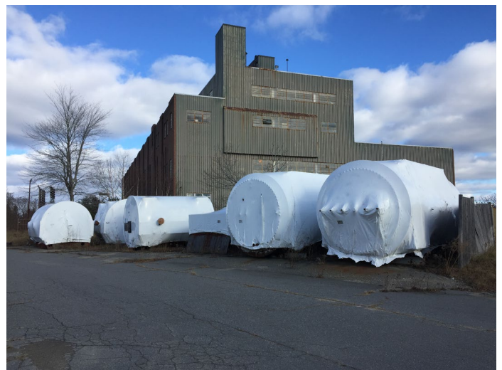
View of wrapped boiler/process equipment, staged outside Powerhouse Building. Wrapped units were not inspected.
