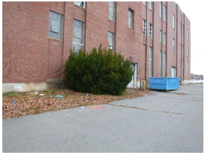
Location of soil boring B303.
