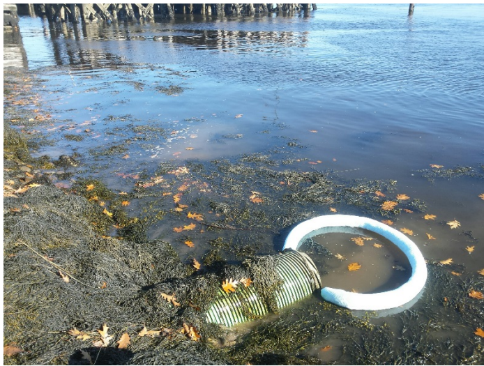
Containment boom at Outfall 006.
