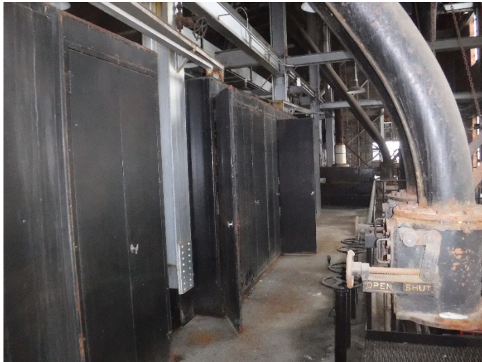
Cabinets in which mercury was reportedly drained, northeastern portion of the Powerhouse interior.
