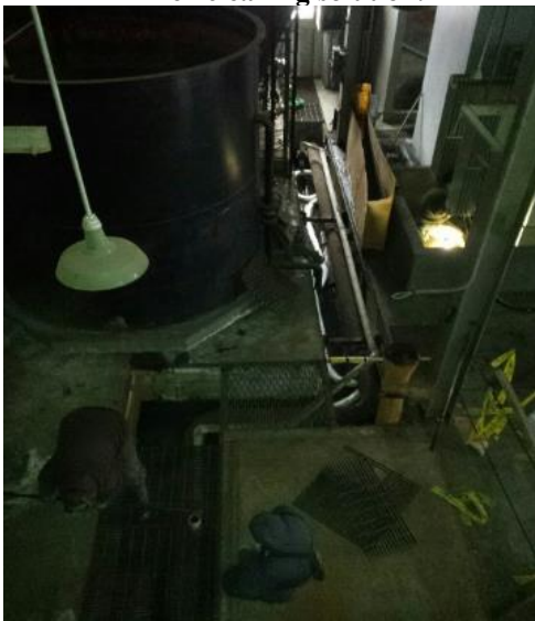
Photo 15: Trench drain network viewed from second floor.
