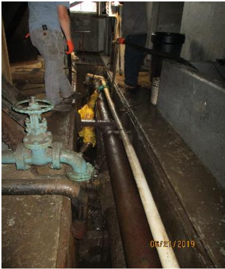
Photo 21: Manually removing sludge from trench drain network.
