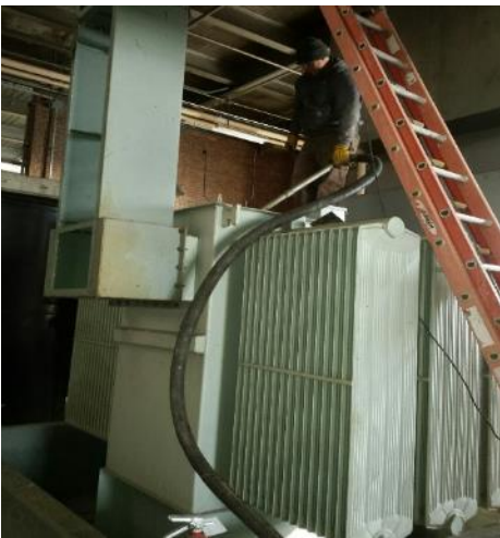
Photo 9: Removing oil from transformer using vector rig.
