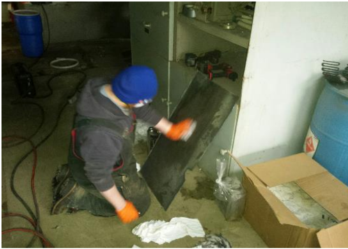
Photo 13: Wiping down cut pieces of transformer with “D-Lime” cleaning solution.
