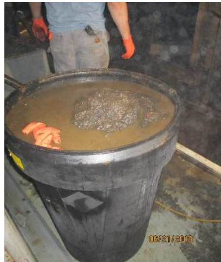
Photo 24: 55-gallon drum of sludge material removed from trenches.
