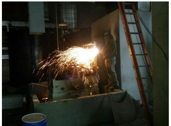
Photo 12: Transformer removal with plasma torch.
