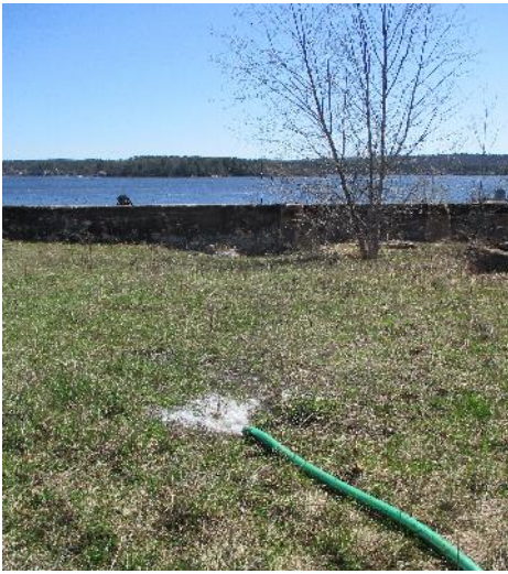
Photo 19: Discharge of treated water to ground surface.
