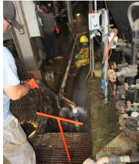
Photo 22: Power washing trench drain network.
