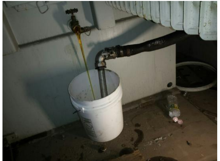
Photo 10: Draining residual oil from bottom of transformer.
