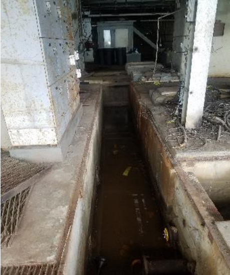
Photo 25: Trench drain system following power wash.
