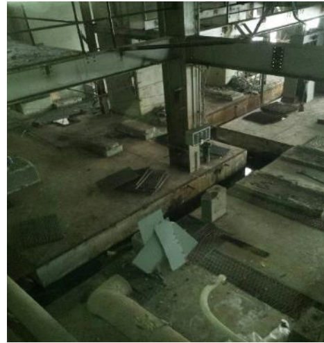
Photo 14: Trench drain network viewed from second floor.
