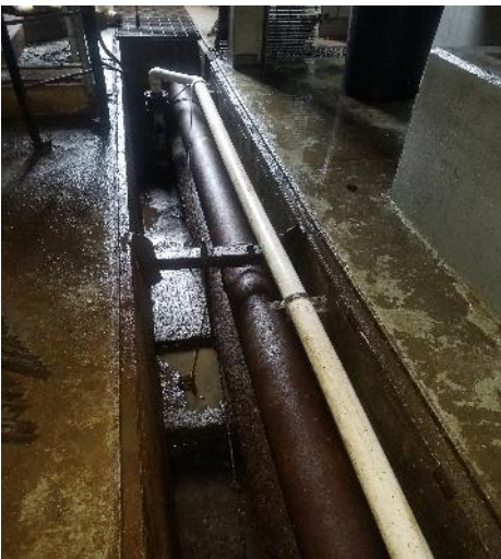
Photo 27: Trench drain system following power wash.
