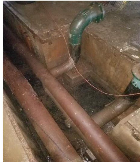
Photo 26: Trench drain system following power wash.
