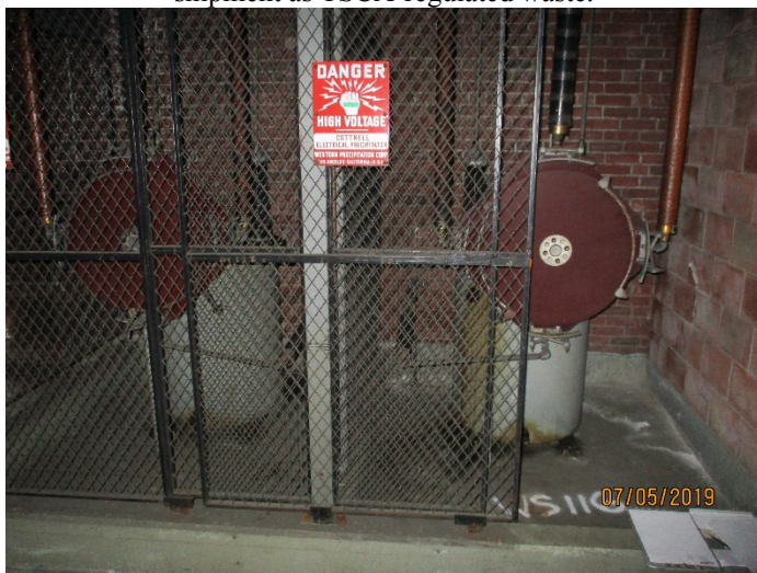
Photo 29: Transformer Serial Numbers 516107 and 516678.
