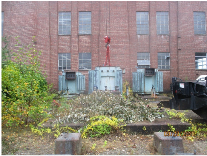
Photo 1: Removal of Transformer No. 28479-1.
