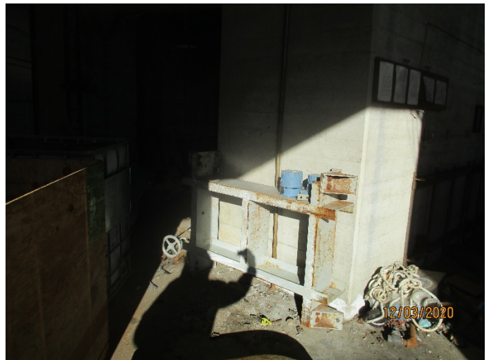
Photo 18: Location of Transformer Serial Number 51336 following removal.
