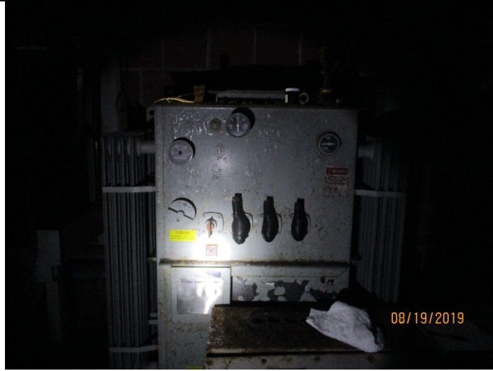
Photo 13: Transformer Serial Number 50539.
