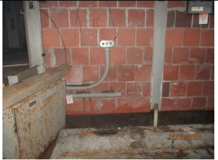
Photo 14: Location of Transformer Serial Number 50539 following removal.
