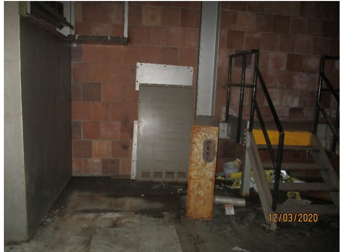
Photo 22: Location of Transformer Serial Number 50541 following removal.
