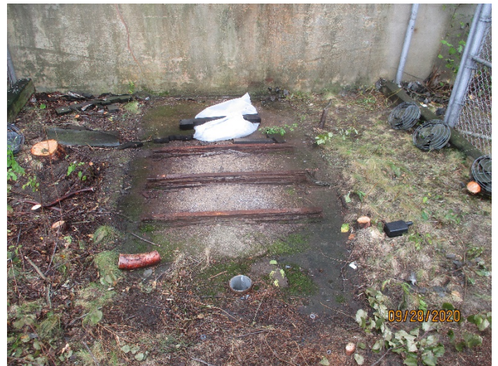
Photo 12: Concrete pad following removal of Transformer No. B363190.
