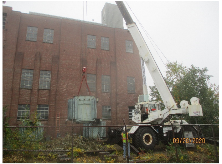
Photo 2: Removal of Transformer No. 28479-1.
