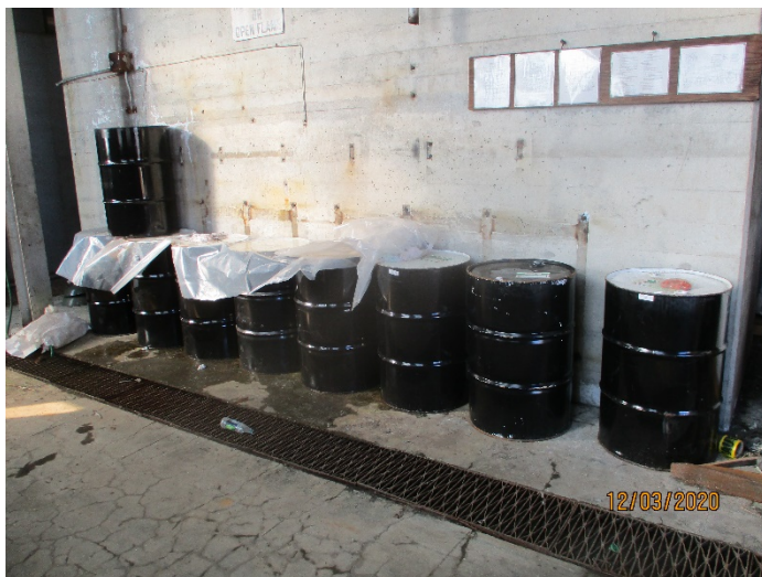
Photo 27: Oily water from spill containment structure, awaiting shipment as TSCA-regulated waste.
