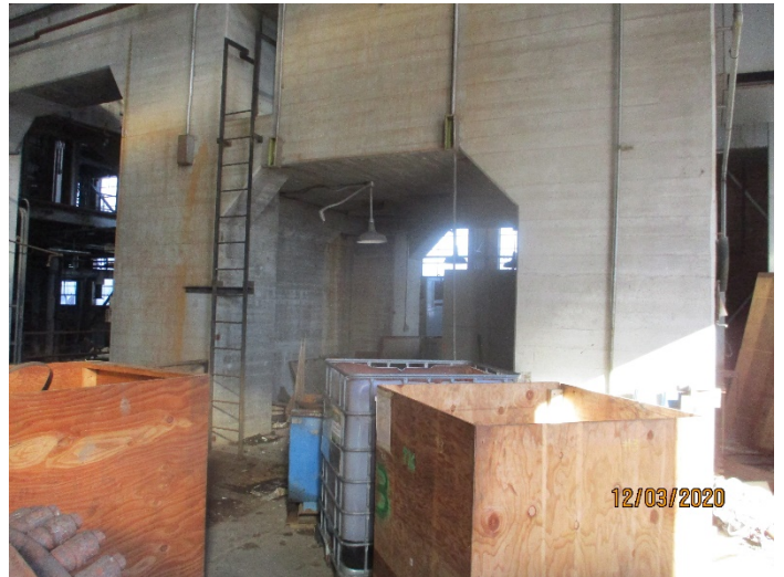
Photo 16: Location of Transformer Serial number 51951 following removal.
