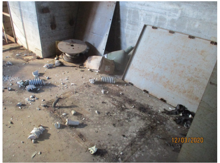
Photo 20: Location of Transformer Serial Number 51337 following removal.
