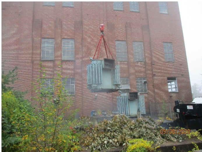
Photo 5: Removal of Transformer No. 28477-1.
