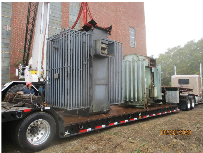
Photo 11: Loading Transformer B-363190 for transport with Transformer 28480-1.
