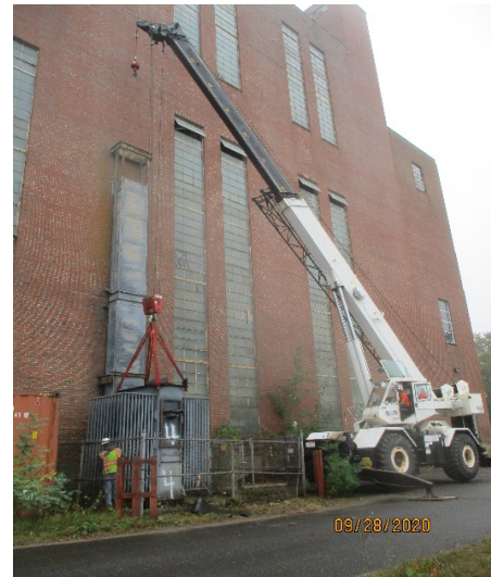
Photo 10: Removal of Transformer No. B-363190.
