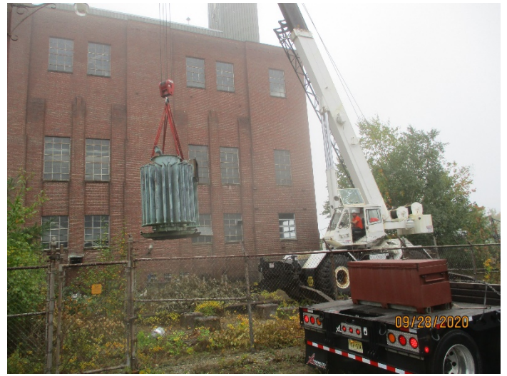
Photo 8: Removal of Transformer No. 28480-1.
