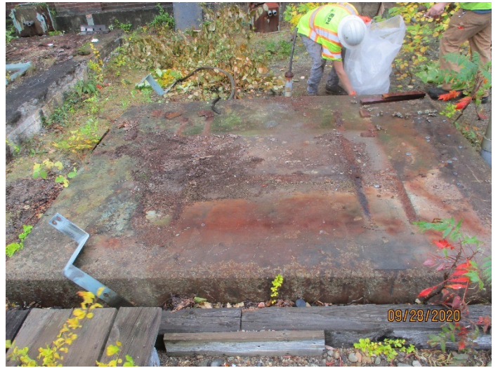
Photo 4: Concrete Pad following removal of Transformer No. 28479-1.
