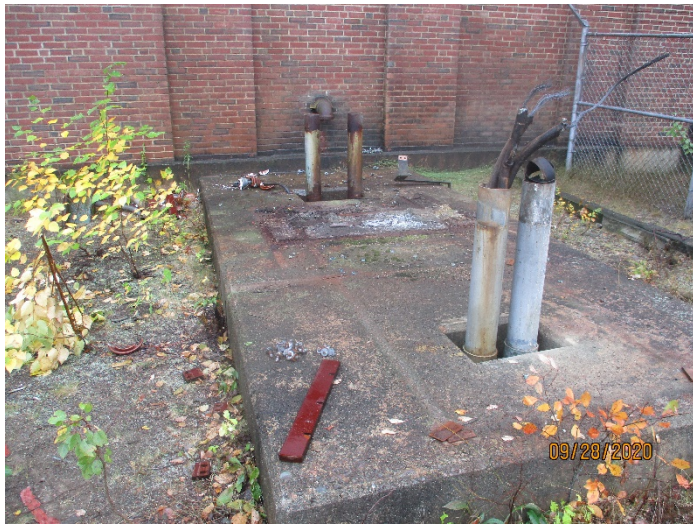
Photo 9: Concrete pad following removal of Transformer No. 28480-1.
