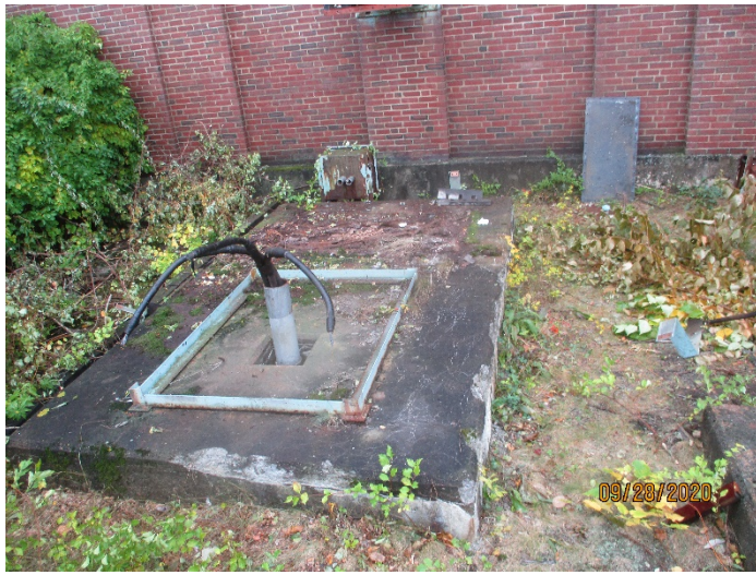
Photo 7: Concrete pad following removal of Transformer No. 28477-1.
