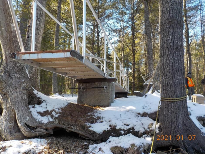
Photo 11: Granite block for gangway
