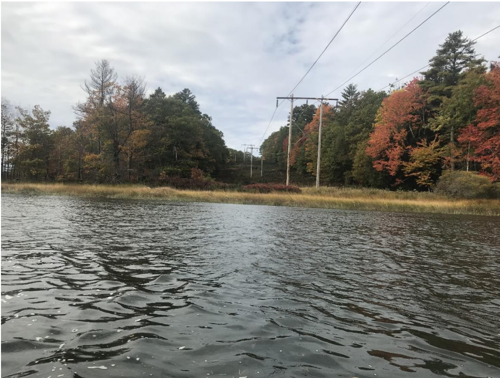
CMP Powerlines, 0.35 mi south of project site
