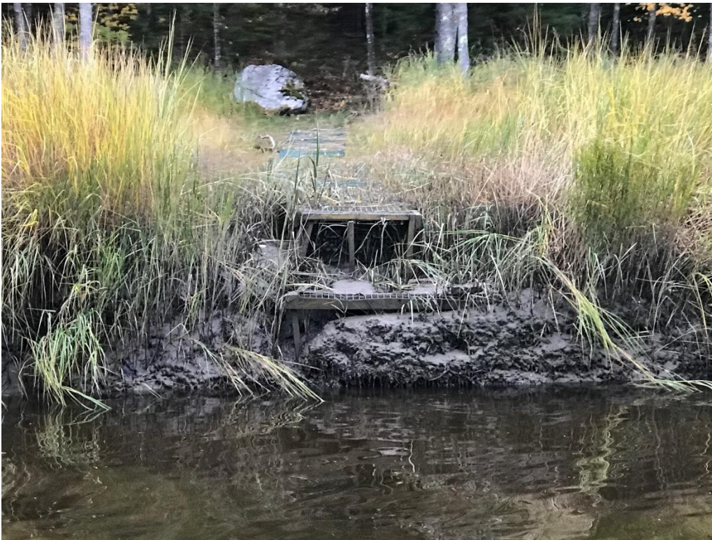
Cheff walkway, 0.7 mi south of project site
