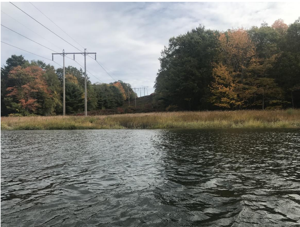
Photo 43: CMP powerline crossing
