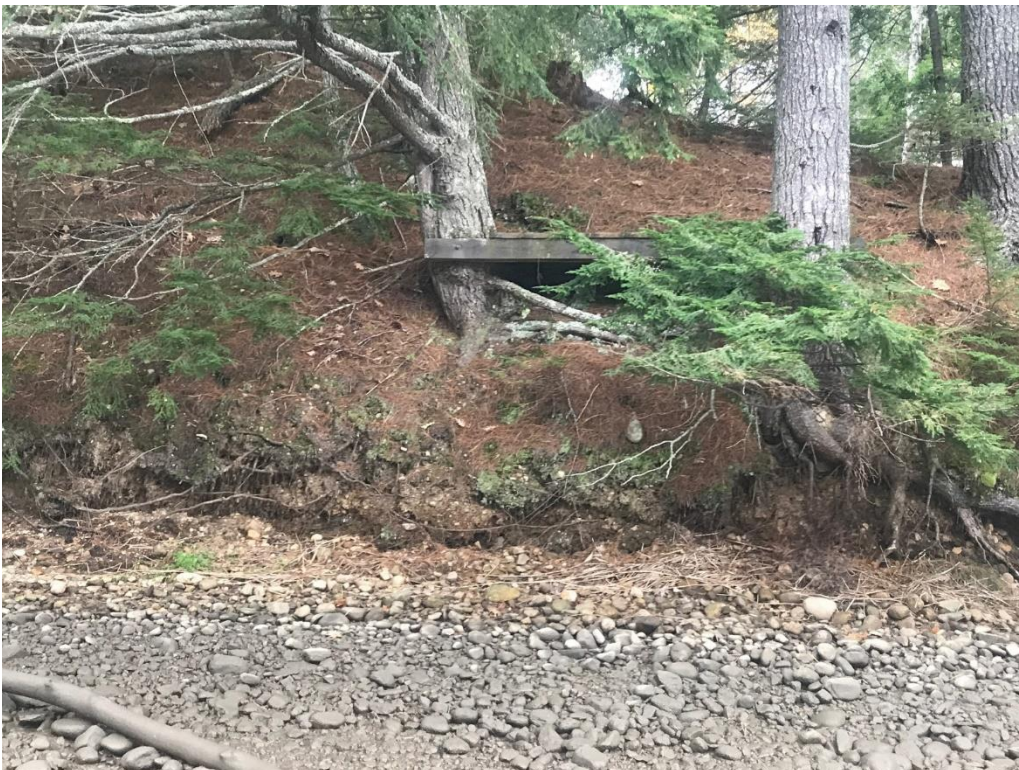
Photo 36: Bolen - unpermitted 'platform' structure adjacent to wetland
