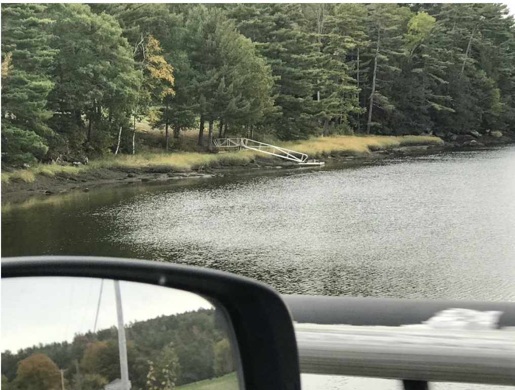
Photo 82: Alum pier, ramp, float
