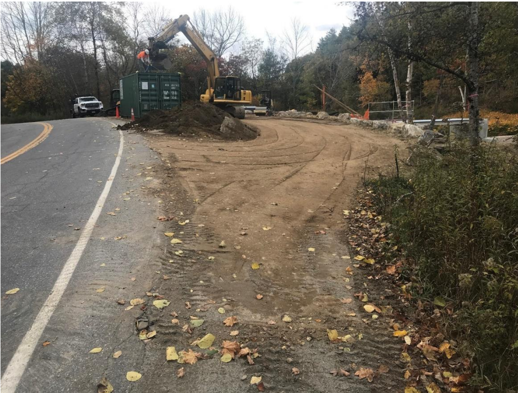
Photo 3: Head Tide Dam, views up and down river, and parking, and stairs. NOT YET COMPLETE
