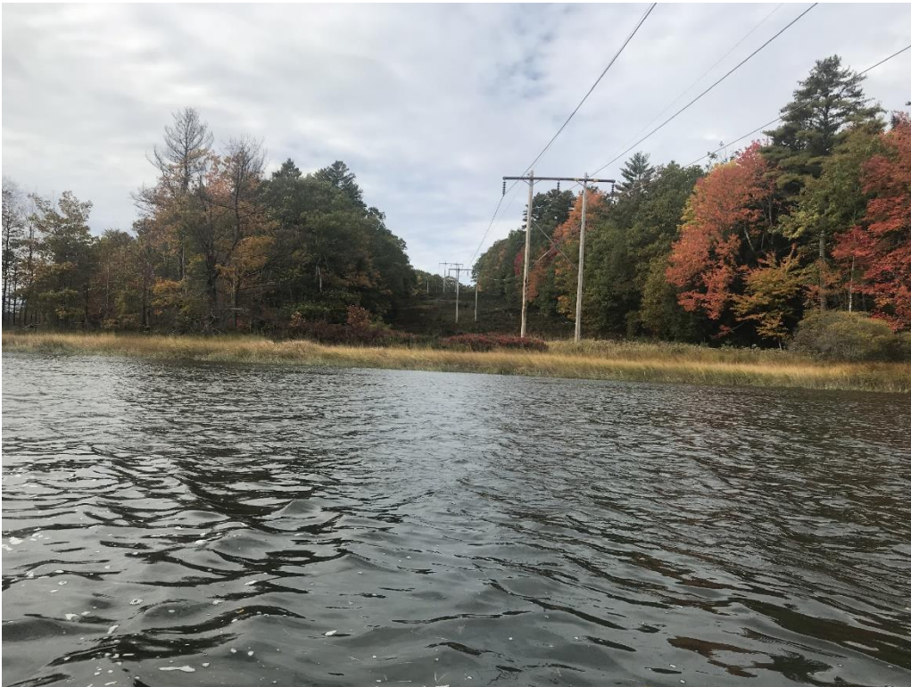
Photo 42: CMP powerline crossing
