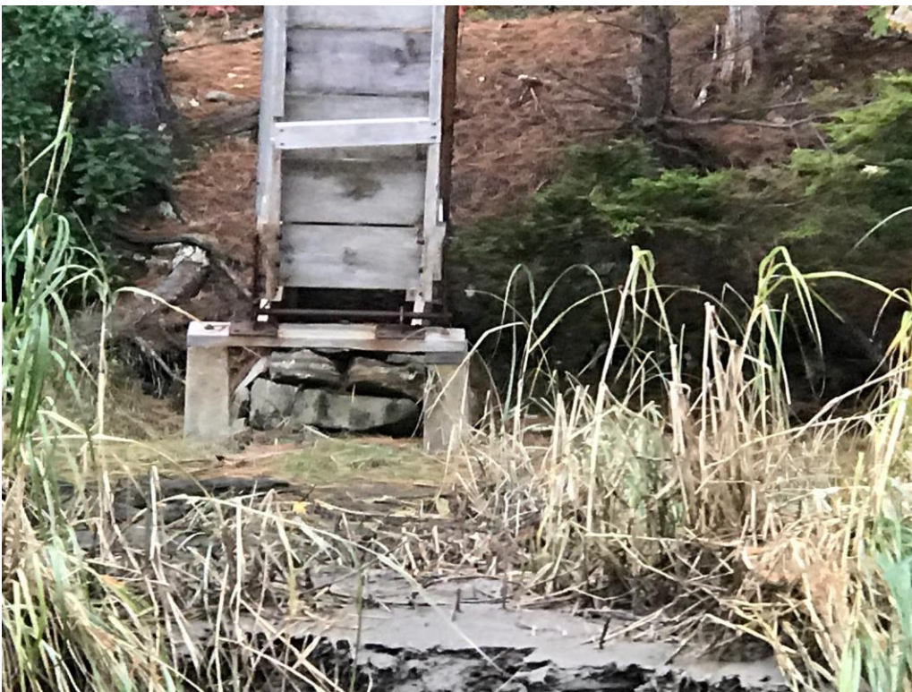
Photo 16: Lifted wooden dock/pier/floats with permanent concrete piers below HAT - (formerly Bill Mook) - Now Leah Sprague - commenter
