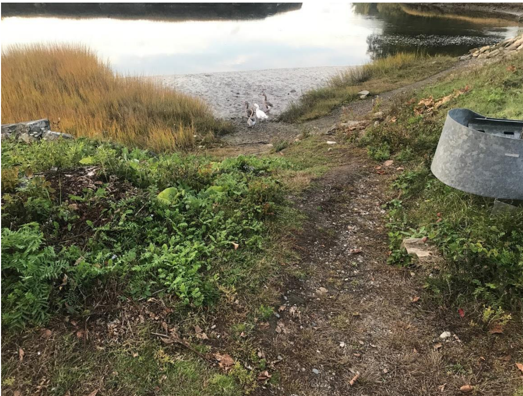
Photo 81: Grange Hall - (private property) being eroded by hand carry use (NRPA permit recently approved to repair)
