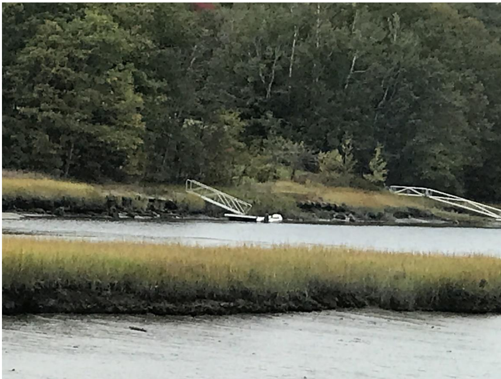
Photo 66: Peele - 8'x12' dock w/ 3'x16' pier, 3'x35' alum ramp & 17' boat (right hand of two shown) - 6/7/16 permitted w/ upland piles
