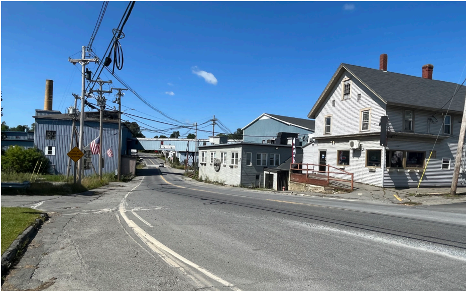
P8 - View looking west from Main Street in Downtown Hartland. The Project will not be visible from this location or anywhere in the downtown village area due to intervening structures, terrain, and vegetation.
