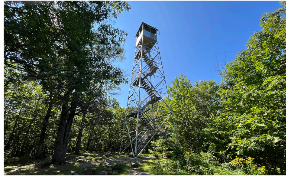
P6 - View looking south toward the Chase Hill Fire Tower at the summit of Chase Hill. The tower is approximately 47 feet in height and allows for 360° views of the surrounding area from the top observation deck.
