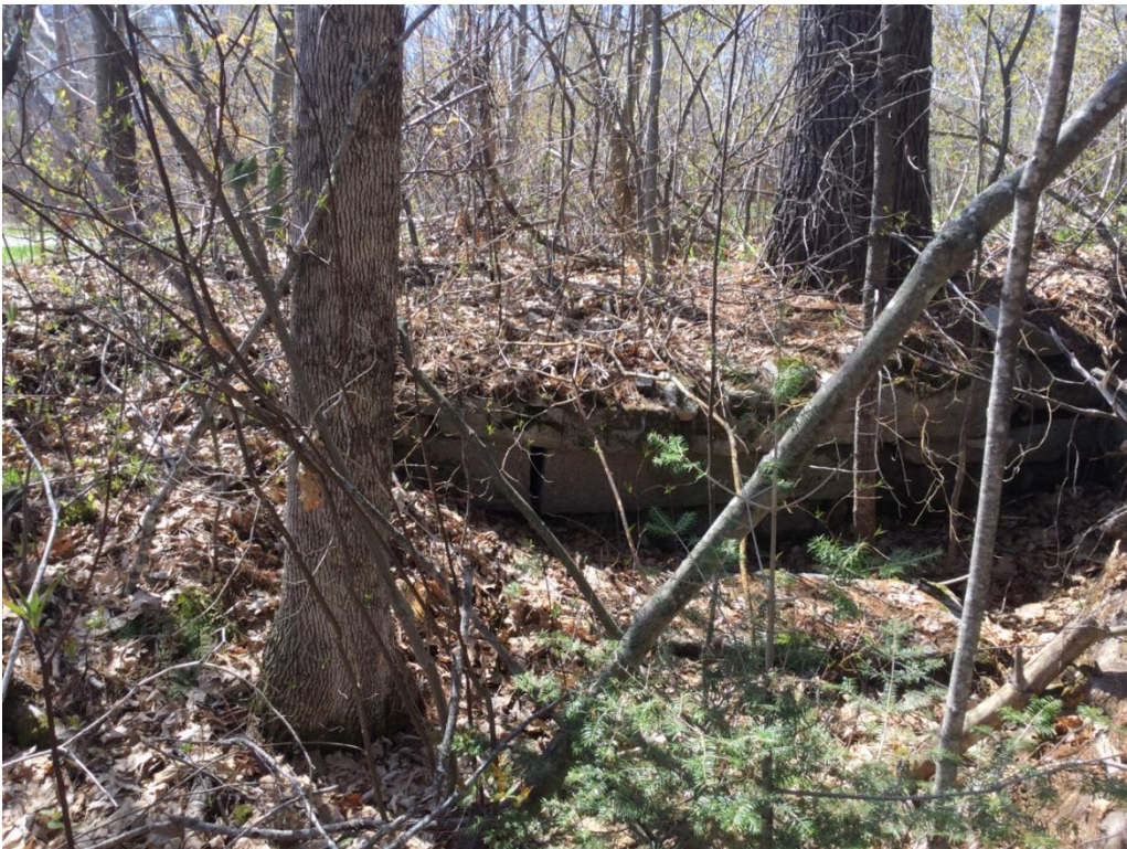
Photo 2. Southwest view of the intact cellar hole wall.
