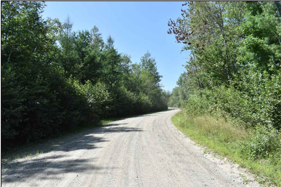
Photo 8. View of the middle of the Project site, facing northwest along Burrill Woods Road.
