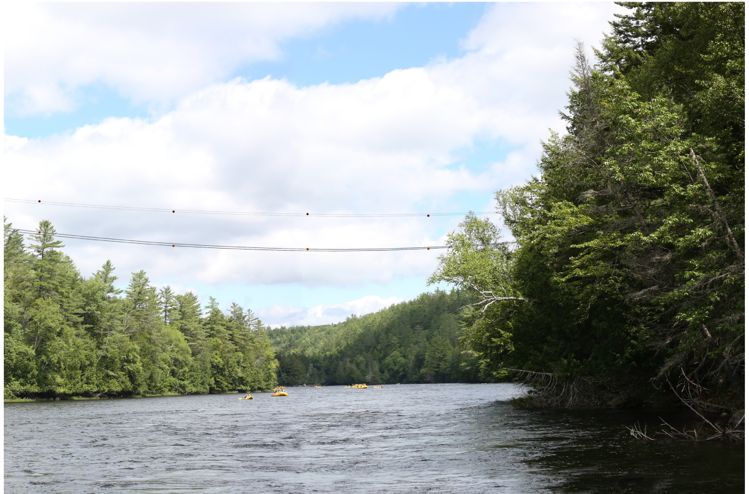
Proposed Conditions: Normal view looking northeast from near the picnic area on the Kennebec River 1,400'+/- south of the proposed HVDC transmission line crossing. The conductors would be approximately 200' above the water level. Approximately eighteen marker balls will be placed on the shield wires and conductors above the Kennebec Gorge.
