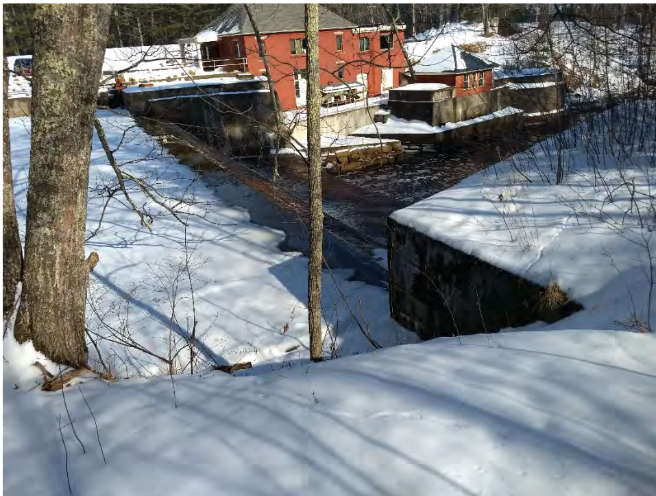
Photo No. 22 – Lower Dam – Upstream side of right abutment.
