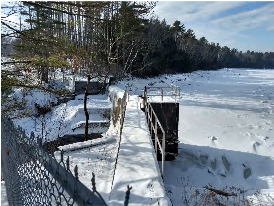
Photo No. 8 – Upper Dam – Dam crest, looking right.
