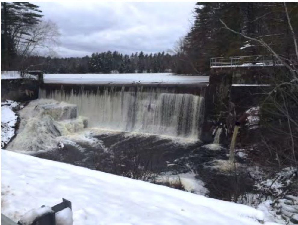
Photo No. 2 – Upper Dam - Site visit in December 2017. Note water over spillway.
