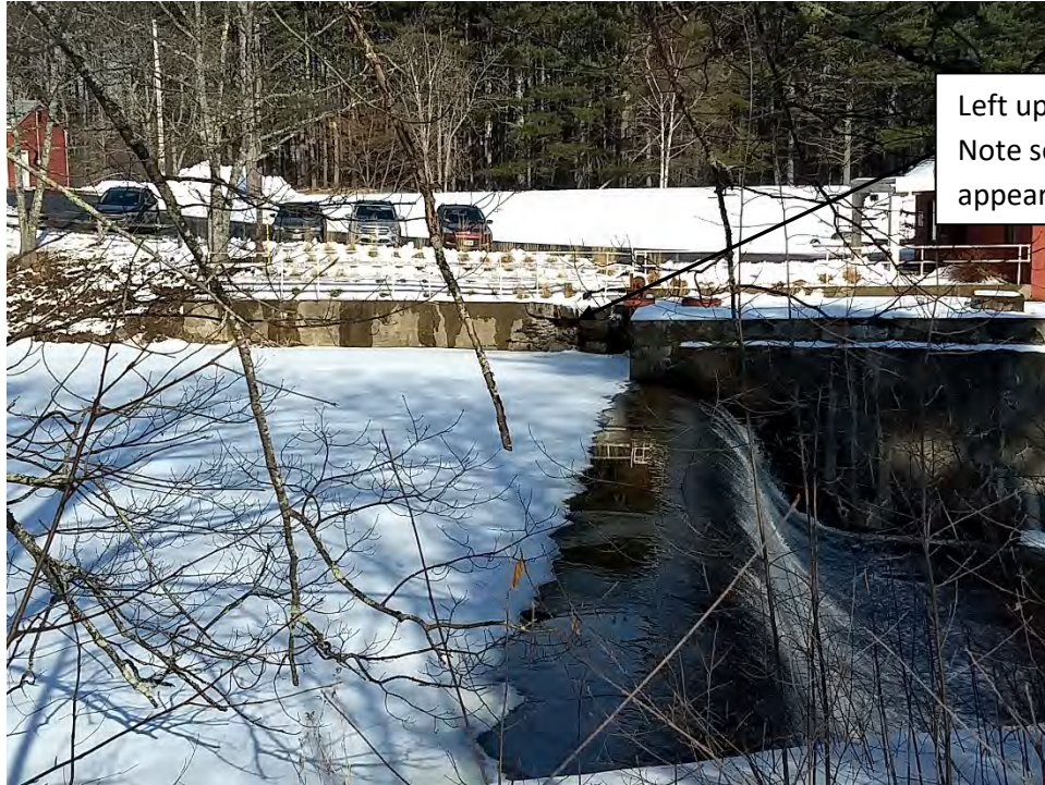
Photo No. 23 – Lower Dam – Upstream left abutment training wall. Note section where concrete facing appears to have failed.
