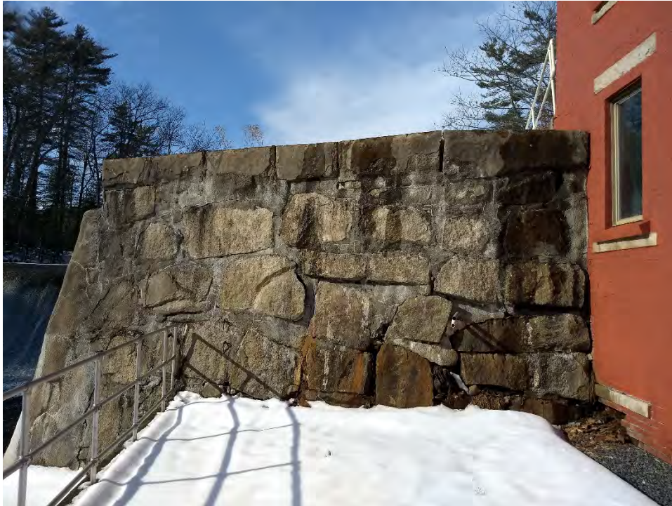
Photo No. 19 – Lower Dam – Downstream side of left abutment.
