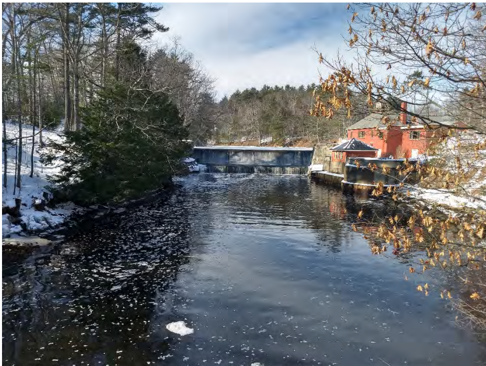
Photo No. 14 – Lower Dam – Downstream side of spillway, looking upstream.
