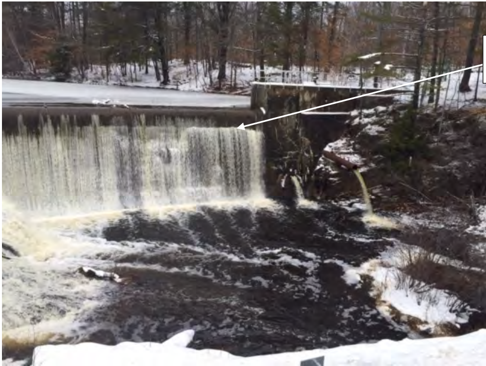
Photo No. 1 – Upper Dam - Site visit in December 2017. Note water over spillway.
