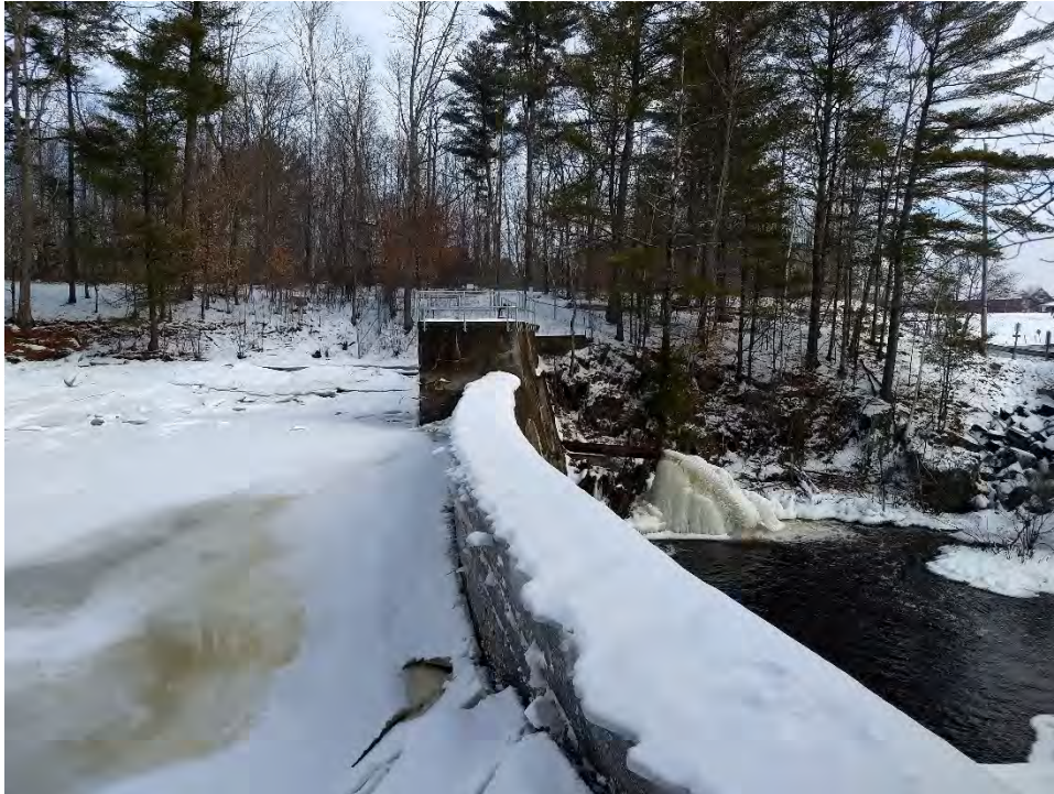
Photo No. 9 – Upper Dam – Spillway sill, looking left.
