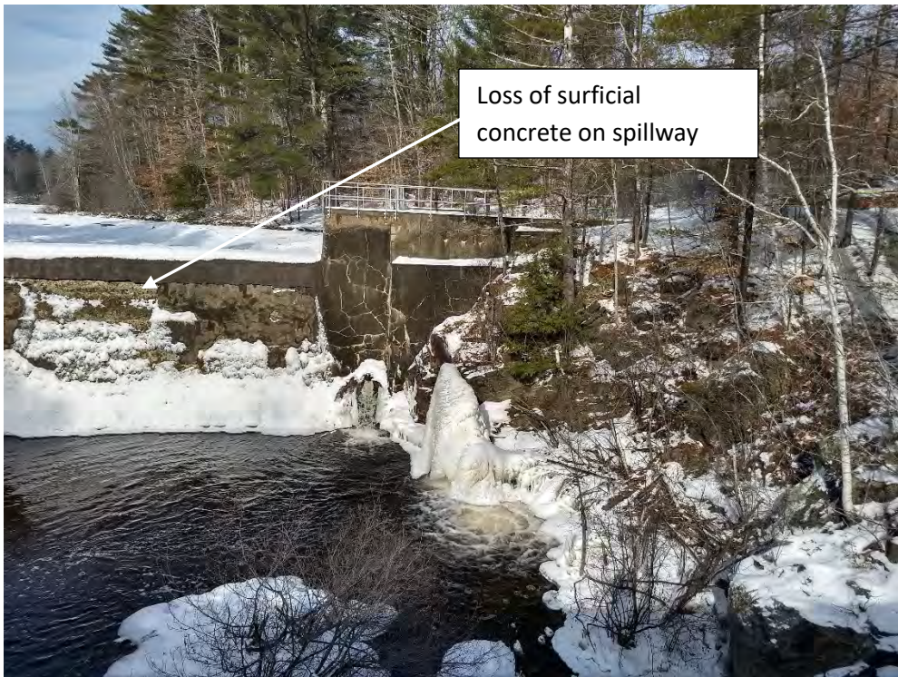
Photo No. 4 – Upper Dam – Downstream side of left abutment and spillway. Note cracks in abutment and loss of surficial concrete on spillway.
