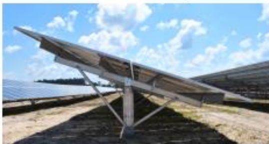
8: Typical solar panel construction (from RBI)
