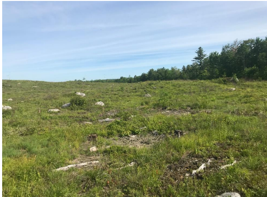
Photo 1: Area 1 cleared field where proposed solar panels will be installed. Photograph taken 6/18/19.
