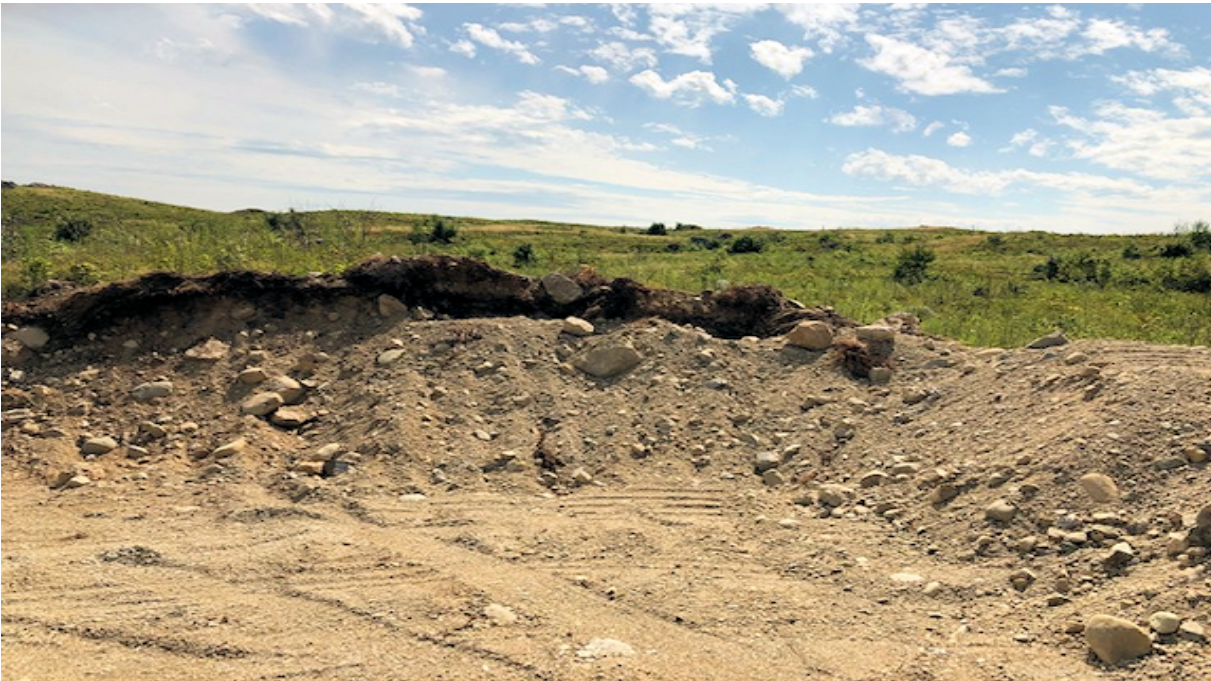
Figure 3. Outwash borrow pit used to extract fill for gravel road.
