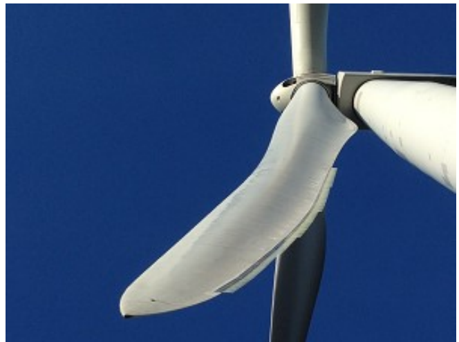
Fig. 1: LNTes at the wind turbine rotor blade
