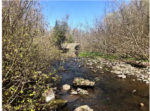
Craig Brook looking upstream at the upper part of the habitat assessment segment, just downstream of the Ingraham Road bridge. Photo: GLEC 2021
