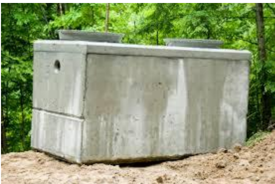
LARGER SEPTIC TANK CAPACITY THAN RQUIRED
