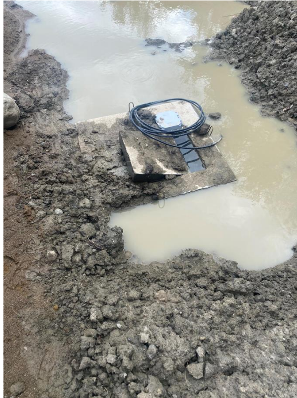
REPAIRING A LEAK IN A SEPTIC TANK OR PUMP STATION
