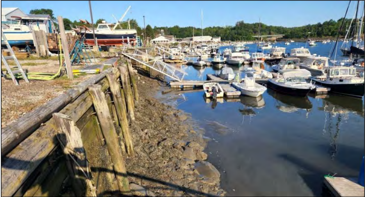
Figure 6-5. Additional view of proposed dredge area, facing west.
