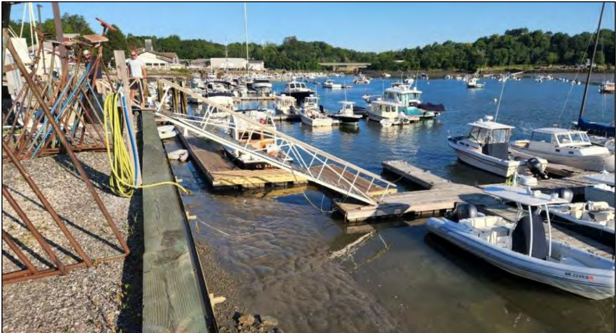
Figure 6-6. Additional view of proposed dredge area, facing west.
