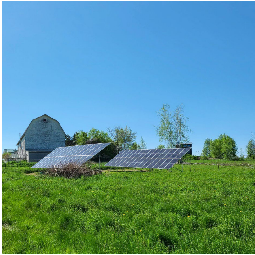
Photo credit: ReVision Energy
