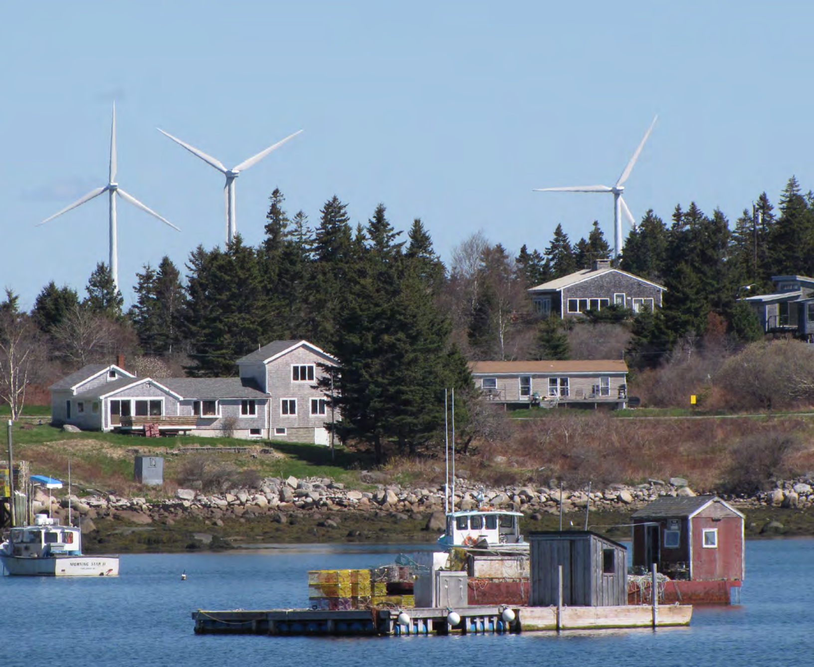
Turbines from Fox Island Wind generate power for the neighboring island communities of Vinalhaven and North Haven.
