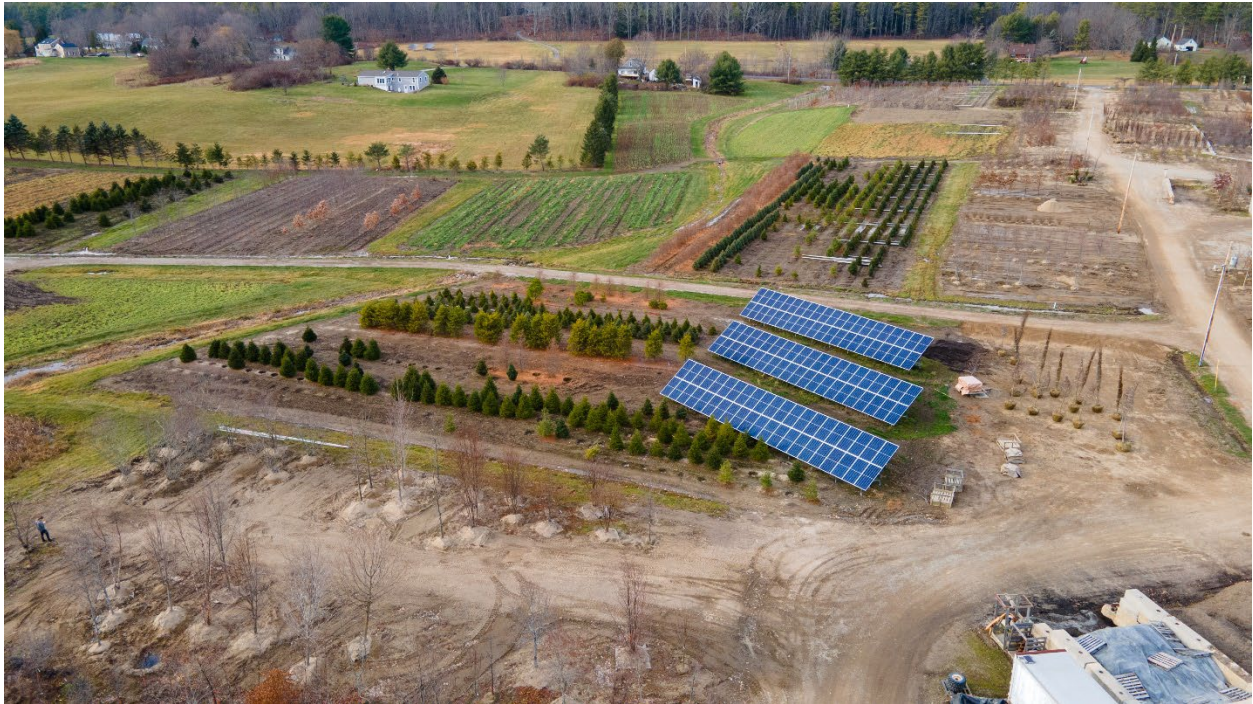
Photo credit: ReVision Energy
