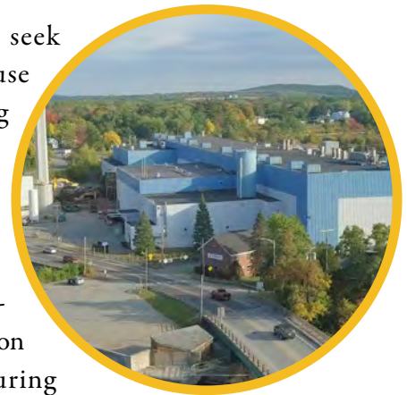
Maine-based startup GoLab is expected to start making climate-friendly wood-fiber insulation in this former Madison paper mill in 2021.
