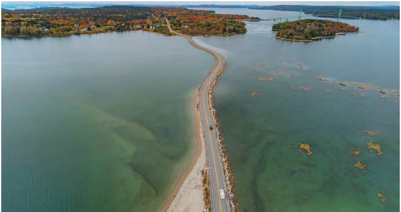
This causeway is a vulnerable portion of the only road that connects the communities of Deer Isle-Stonington to the mainland. Yet with increasing severity of storm surge and rising seas, this vital transportation link is threatened.
