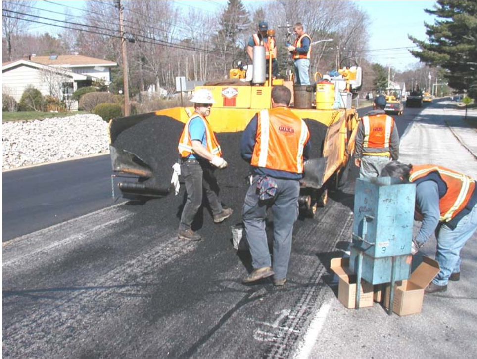
Paving Inspector loads the Quartermaster splitter.
