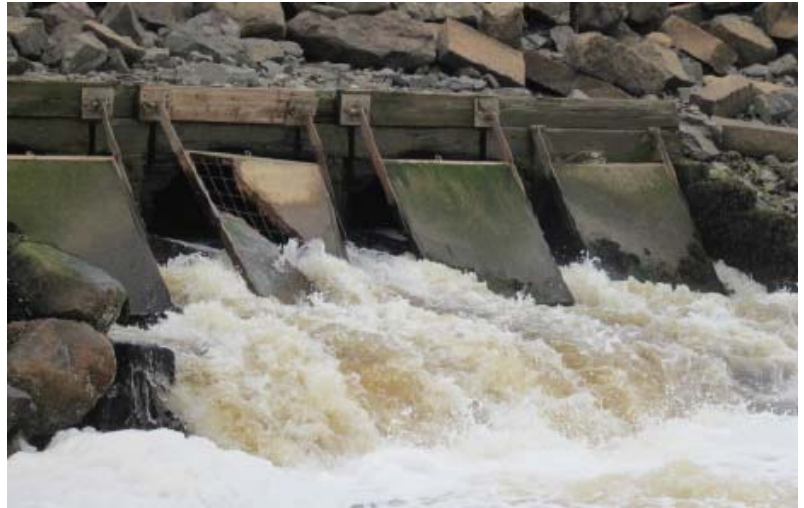
Photo 2. Dyke Bridge culverts with flap gates.
