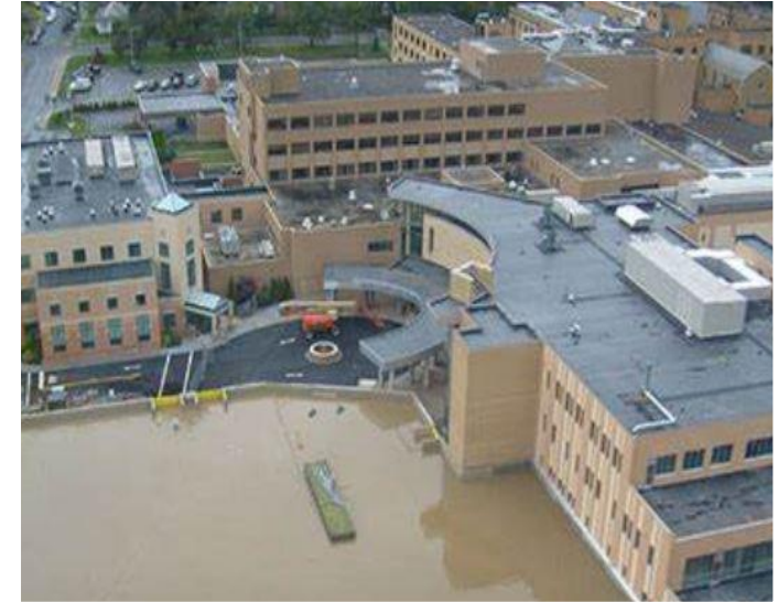
Constructing floodwalls around damaged facilities.
