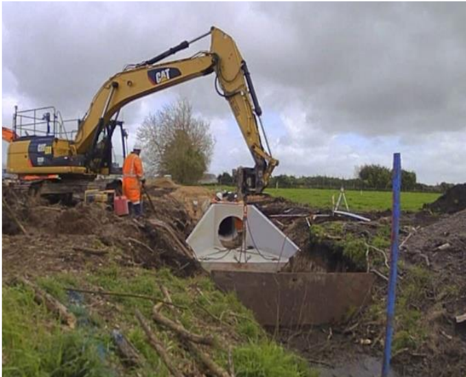
Installing new drainage facilities (including culverts across a damaged road).
